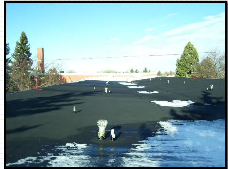
Lewis & Clark Elementary Reroof
