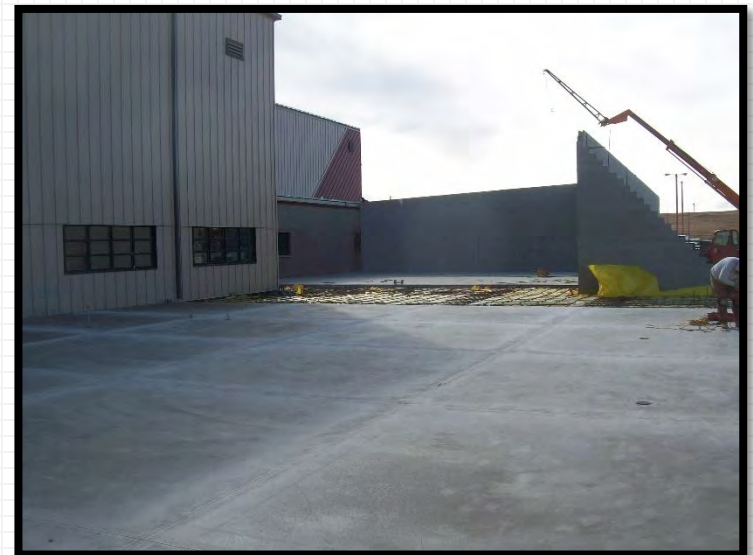
Browning Vocational Technology Building
